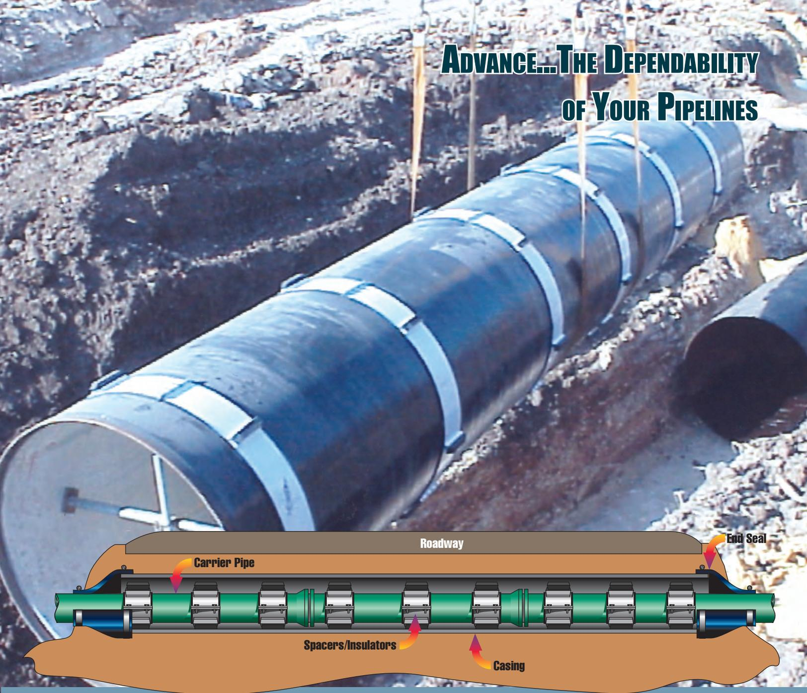
Advance Products & Systems' Casing Spacers and Insulators combine proven dependability and ease of installation to outperform the labor intensive, inefficient and unreliable wooden skids. APS Casing Spacers and Insulators are your answer to lower installation costs with continued access for maintenance.
