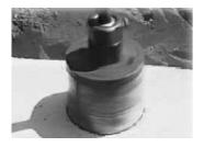
STEP 1 Make sure bit is perpendicular to mainline. Core the proper size hole. Feel inside hole and clear any remaining material.
