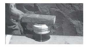
STEP 5 Place the 2x4 board onto the top of the PVC hub adapter
