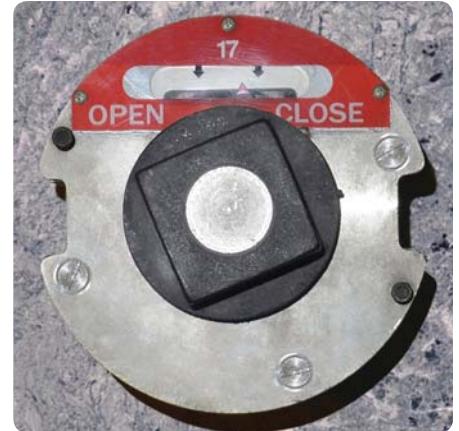
Precise position of valve is difficult to determine.
