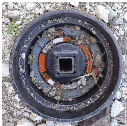
The two simulations above show how dirt and debris can accumulate on the Position Indicator WITHOUT a Debris Shield.
