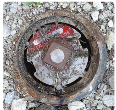
The two simulations above show how dirt and debris can accumulate on the Position Indicator WITHOUT a Debris Shield.
